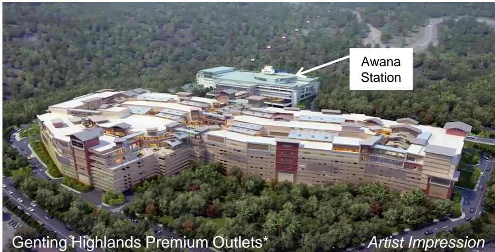
Awana SkyWay Cable Car system
